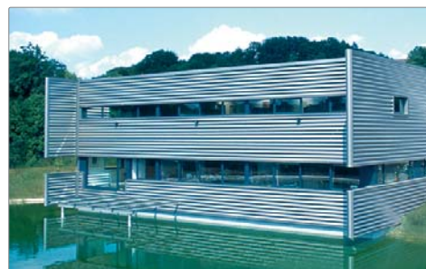
interscience R&D center and manufacturing plant Mourjou FRANCE
